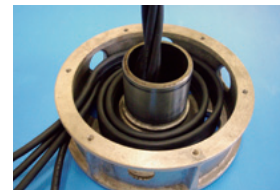
Small space wiring of twisting shaft
